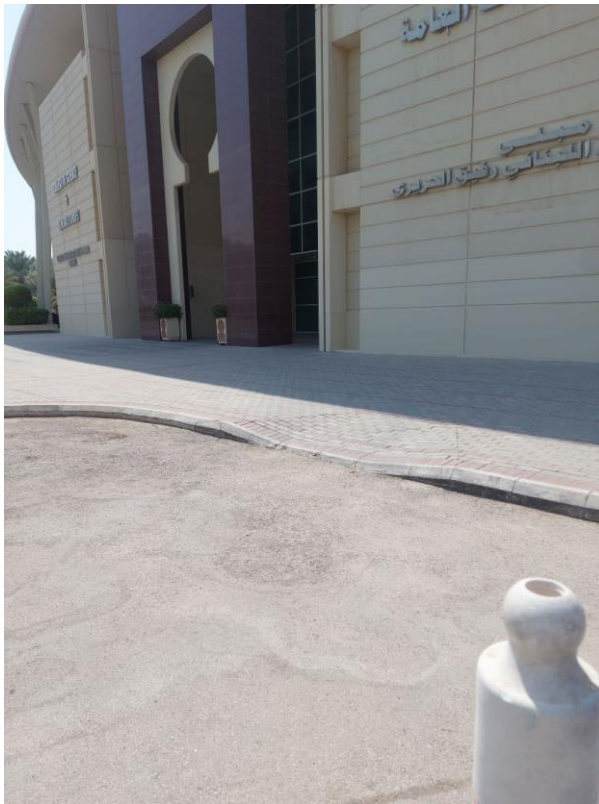
Ramp @ Building's entrance
