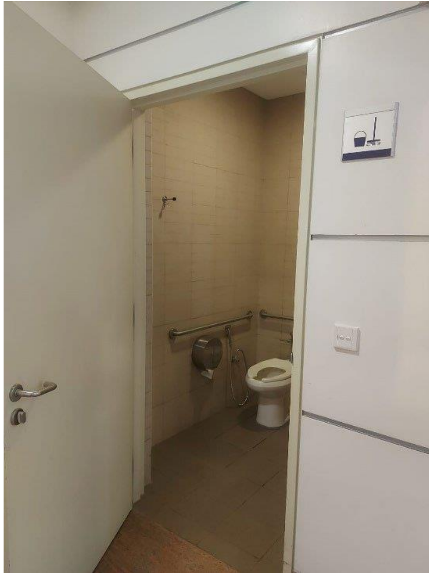
Fully fitted accessible toilet
