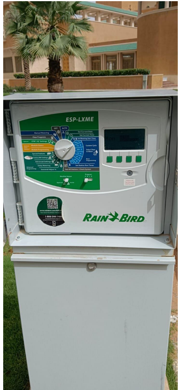
Irrigation Controller
